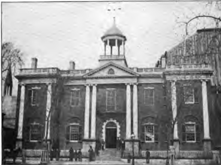
OLD COURT HOUSE, PORTLAND, BUILT 1816.
